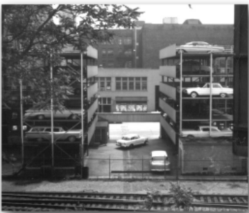
View of the Pigeon Hole Parking from Wood Street, 1961.
